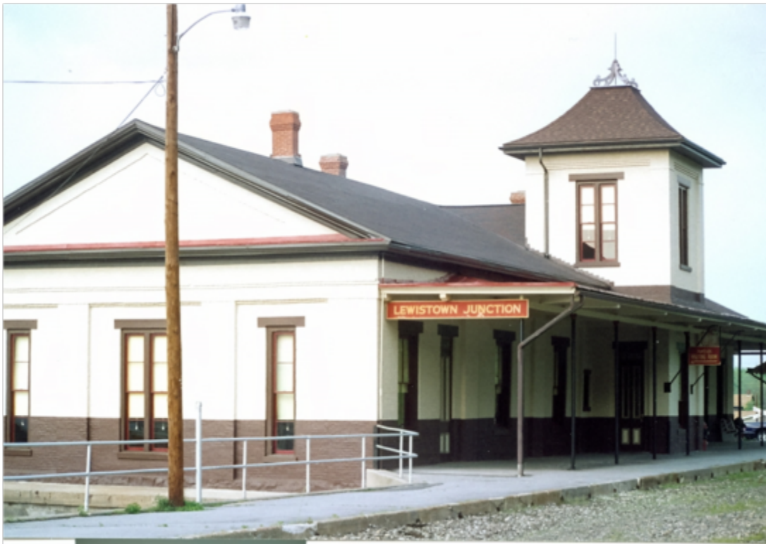
Lewistown station after restoration
